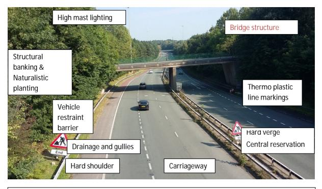
Typically a Bridge Structure –includes, waterproofing, deck, retaining wall, bearings, expansion joints, parapets,
